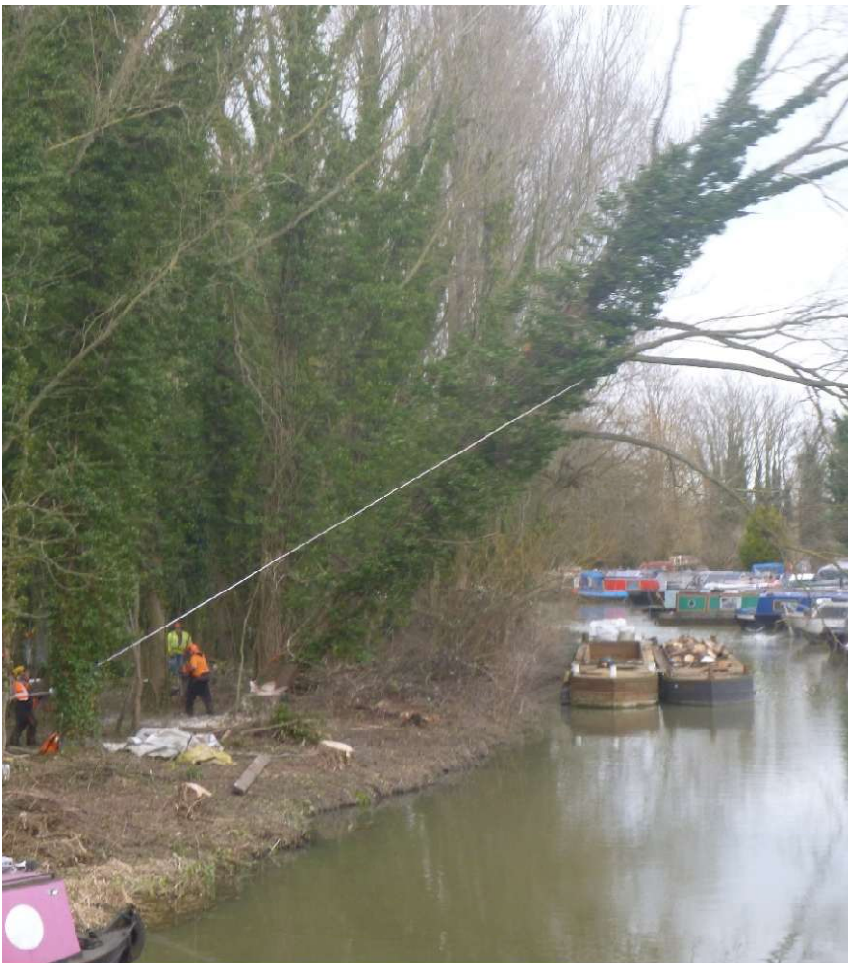
Timber! [Photo: Steve Morley]
