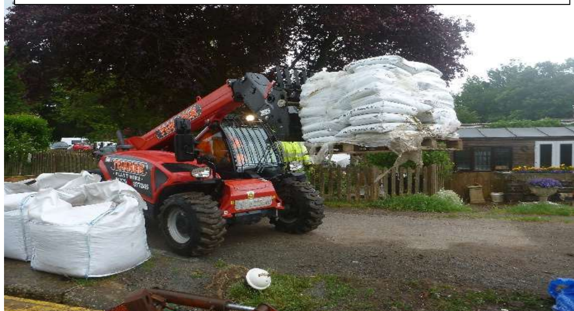
Bentonite delivery [Photo: Steve Morley]
