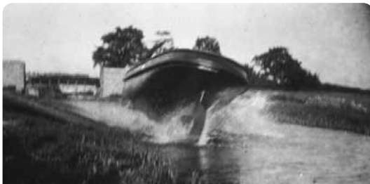
Creating a splash! Launching a tug sideways into the Buckingham Arm. © Unknown
