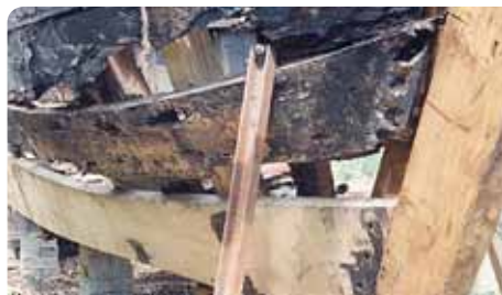
New stempost and planking © Rickmansworth Waterways Trust
