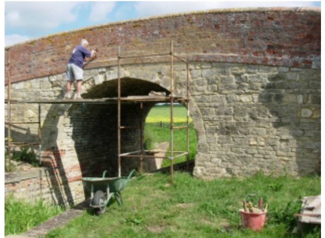
Restoration work going well on the bridge at Little Hill Farm
