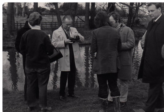
An inspection of the Buckingham Canal in 1973.
