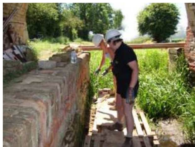
Volunteers working on bridge at Little Hill Farm
