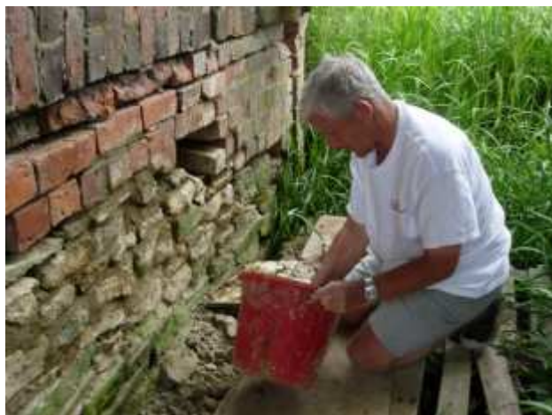
Nigel Preston re-pointing bridge at Little Hill Farm
