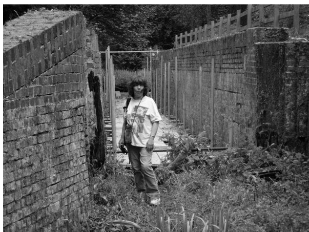
PROGRESS MADE SO FAR AT THE SITE
